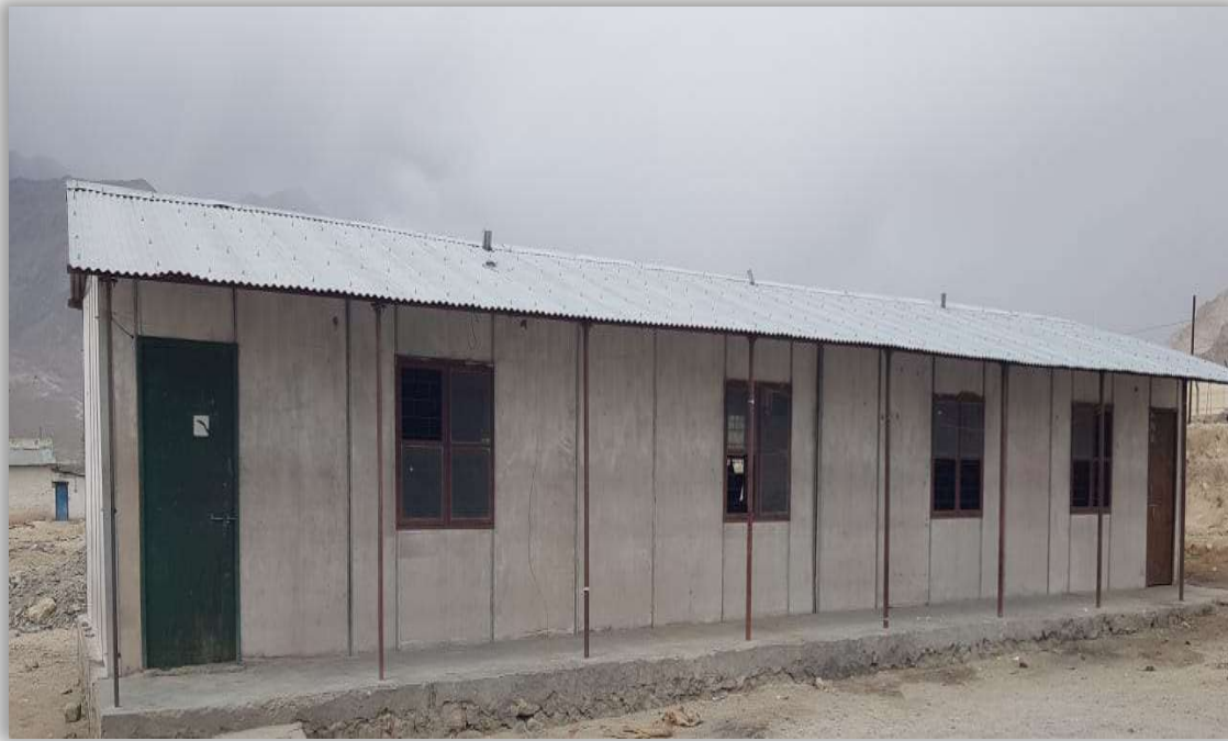
Khaltse, Western Ladakh
